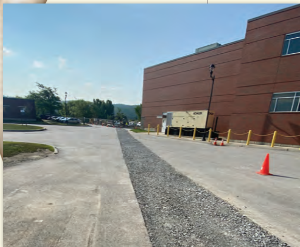
The long trench crossing a large section of the Northwest Medical Center access road and parking lot.
