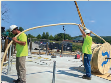
470' of 1-1/2" MediTrac ® being run through the non-metallic conduit.
