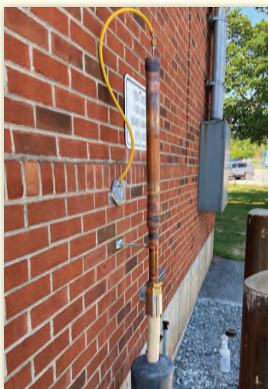
1-1/2" MediTrac ® fitting with a pre-brazed test setup ready for testing.
